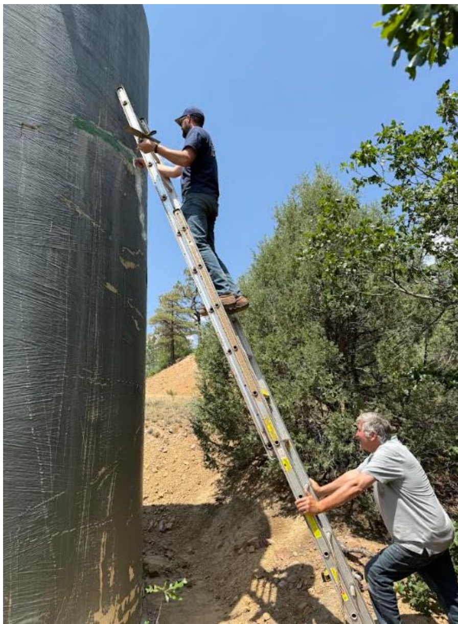
Leak Repair on Ponderosa Tanks
